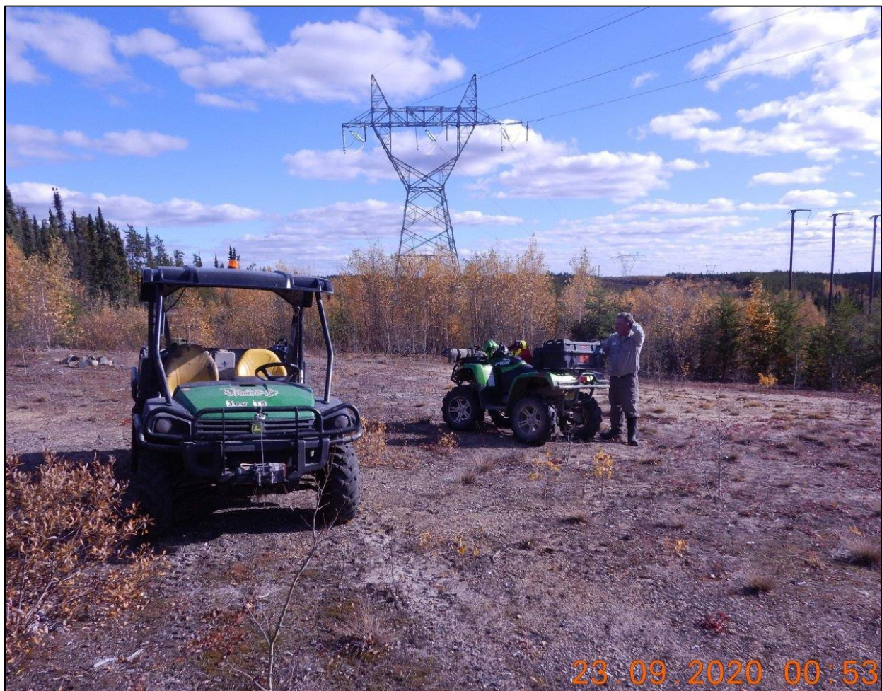
FIGURE 5.5 POWER LINE AT TOWER LAKE
